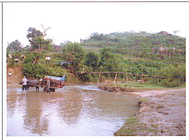
Picture 2: From upstream
