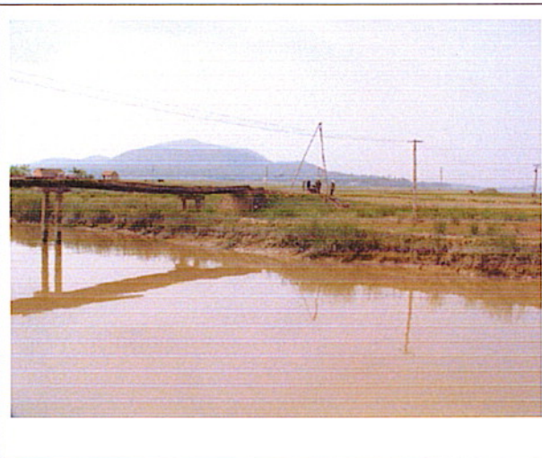
Picture 1: The existing bridge from upstream
