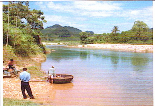
Picture 2: From down stream. On right bank abutment of former bridge (washed Away) is seen.
