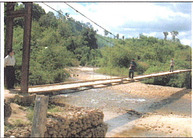
Picture 2: From upstream
