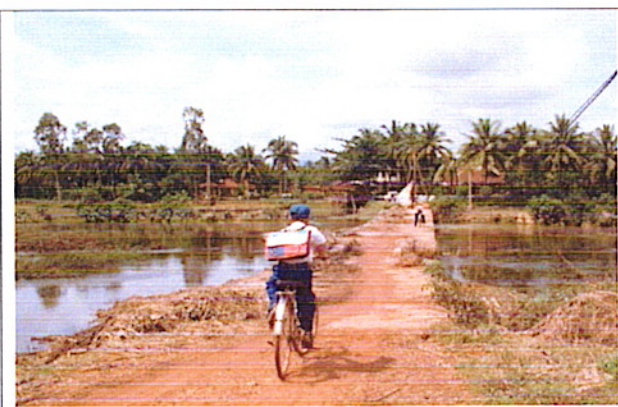
Picture 1: On bridge center line from right bank.
