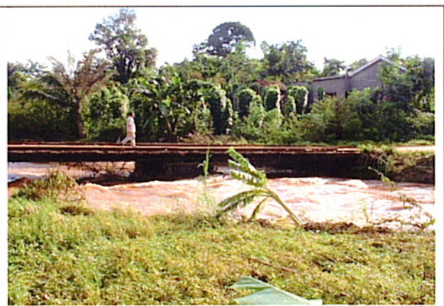
Picture 2: Existing Bridge
