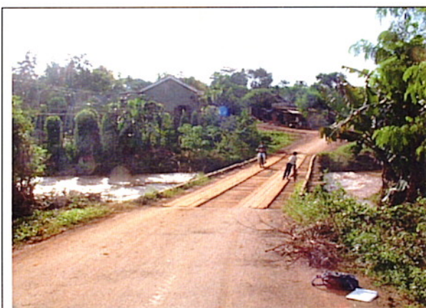
Picture 1: Existing Bridge
