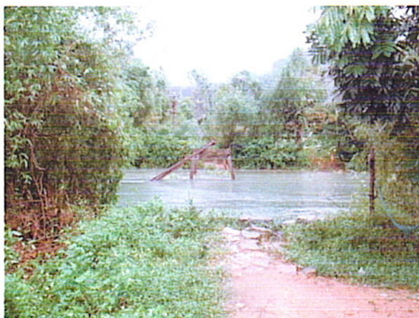
Picture 1: The former bridge from left bank in front of school
