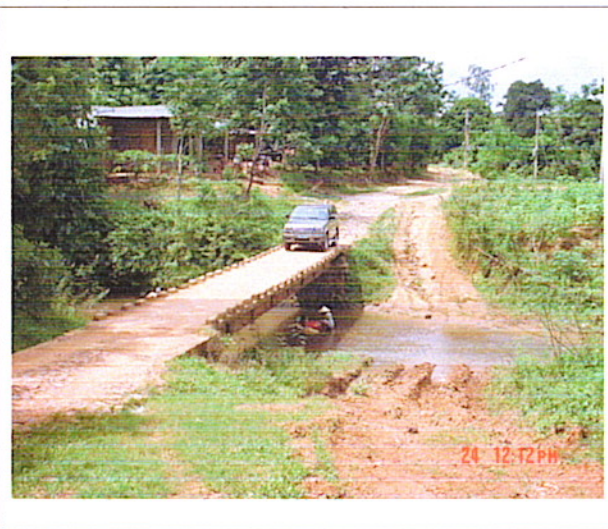
Picture 1: The existing bridge from right bank
