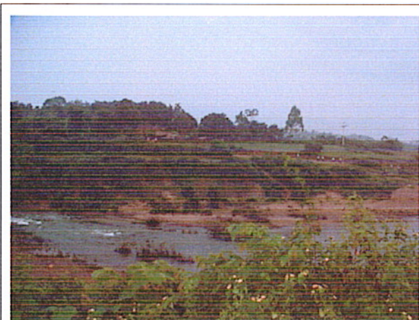
Picture 1: The proposed bridge alignment from high flat area of left bank
