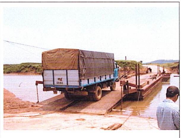
Picture 2: The existing pontoon bridge from right bank
