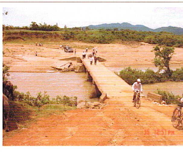
Picture 2: The existing bridge from left bank
