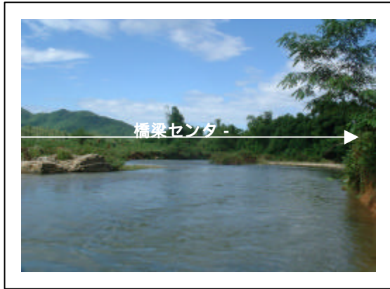
写真 - 3 NO.27 Hoi Phuoc 橋(Da Nang City)
