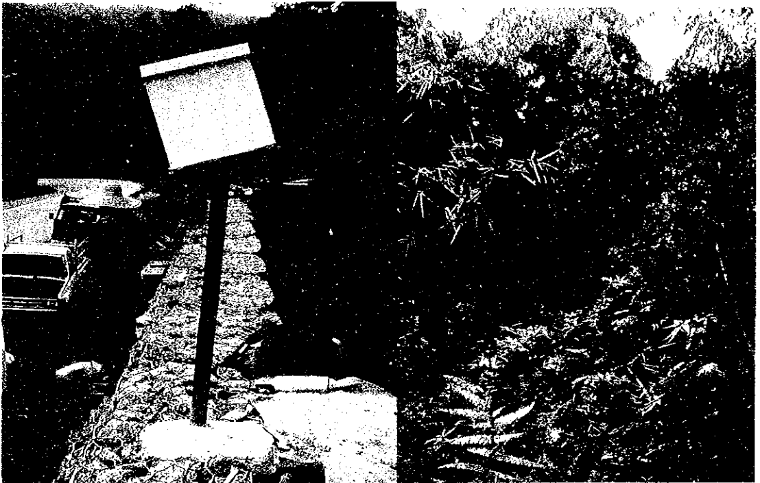
Figure 3.5.30 Wire Extensometer (81.33km Lower)
