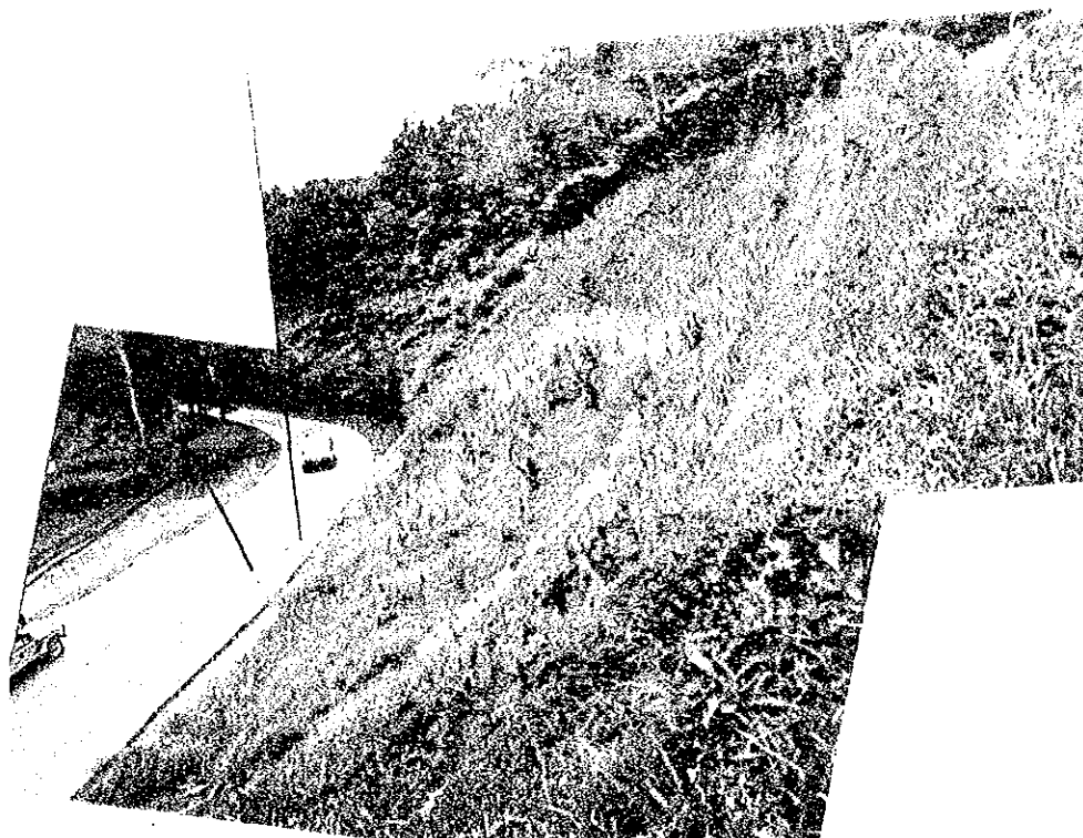
Figure 2.6.2 Earthwork (Soil Cutting)
