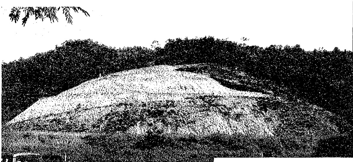
Figure 2.6.1 Earthwork (Counterweight Embankment)
