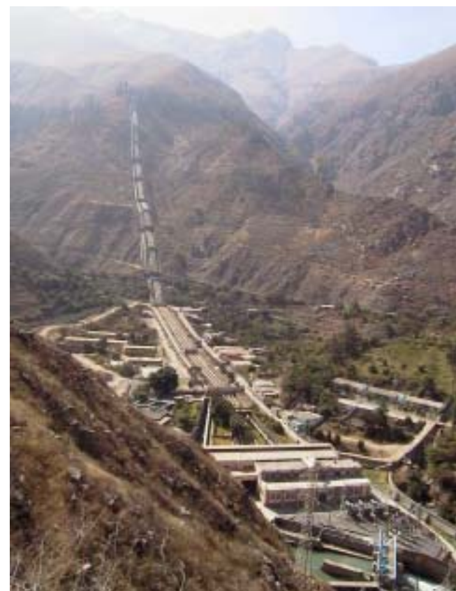
Callahuanca Hydro-electric Power Station: Excess water is discharged into the Santa Eulalia River
