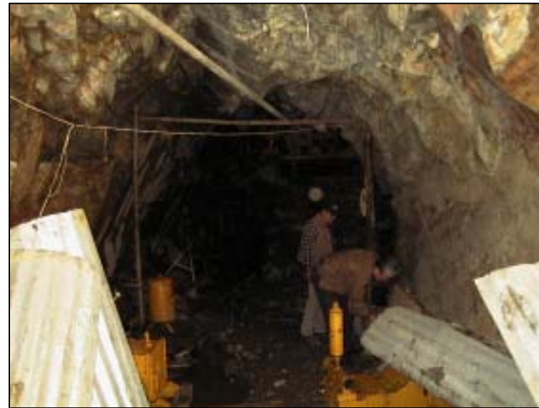
Morro de Arica Dam Site-2: Test adit
