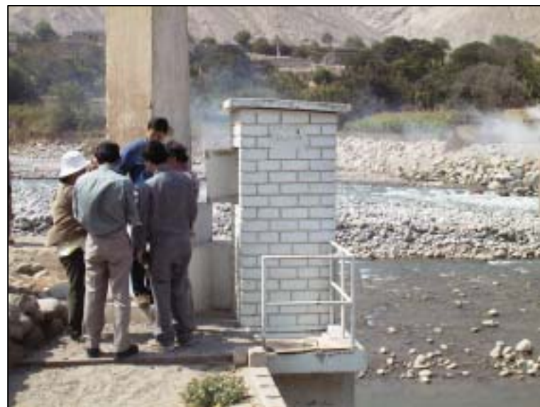
Sosci Gauging Station
