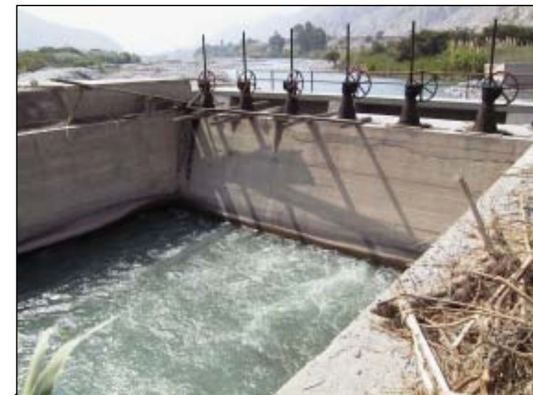
Irrigation Sluice Gate at New Imperial
