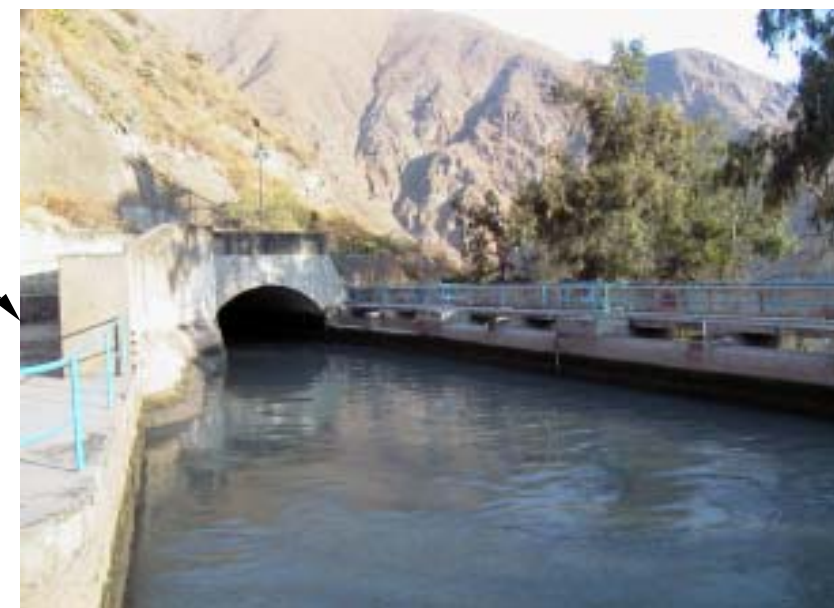
Tunnel Outlet from Matucana Hydroelectric Power Station at the Connection Pond for Callahuanca Power Station
