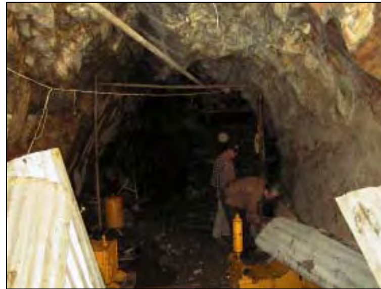
Morro de Arica Dam Site-2: Test adit
