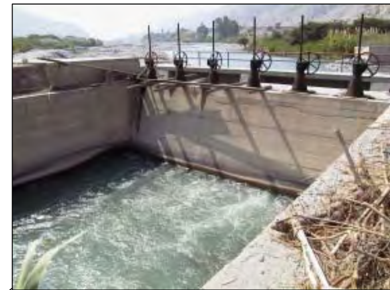
Irrigation Sluice Gate at New Imperial
