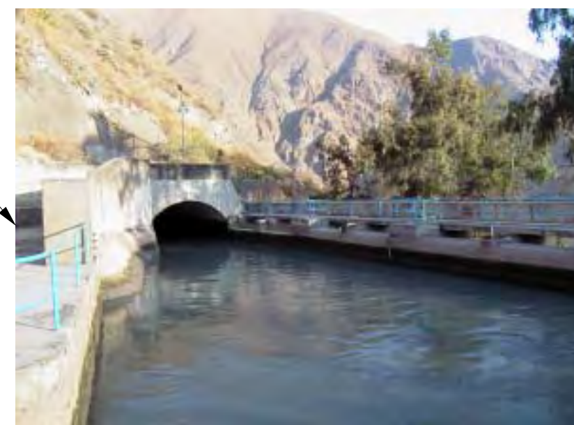
Tunnel Outlet from Matucana Hydroelectric Power Station at the Connection Pond for Callahuanca Power Station
