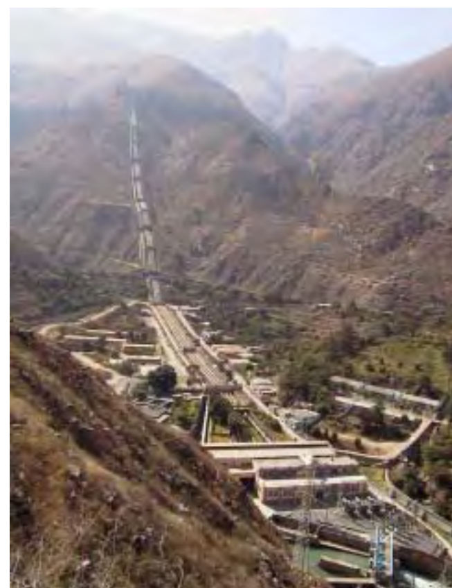
Callahuanca Hydro-electric Power Station: Excess water is discharged into the Santa Eulalia River
