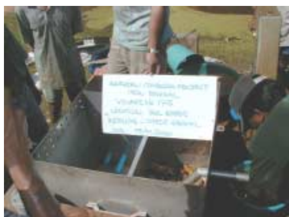
5. Filling coarse gravel into D chamber
