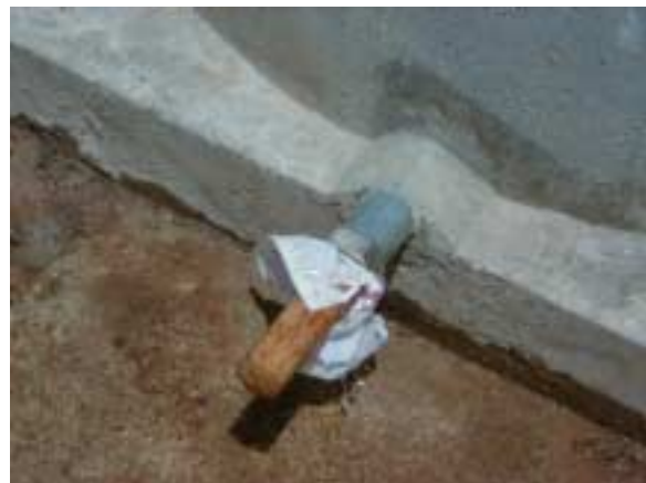
12. Wooden plug installed by villager
