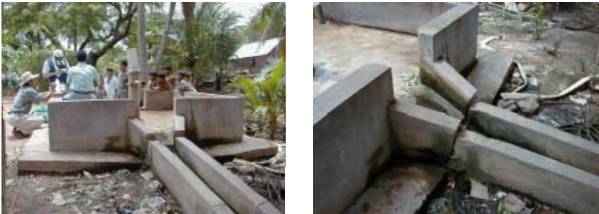
Figure 2.8 Crack in the Drain
