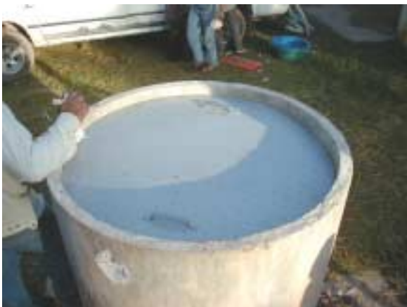
11. Installation PVC perforated plate for IRD
