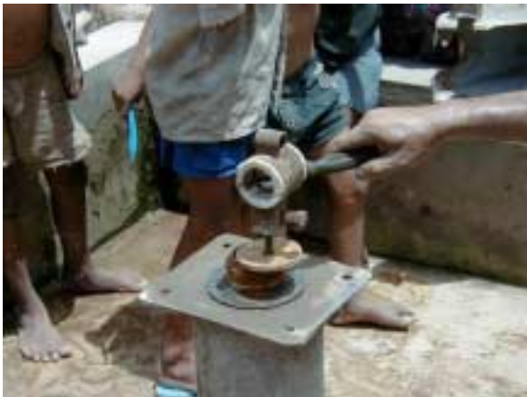
7. Longer pump rod at No.181
