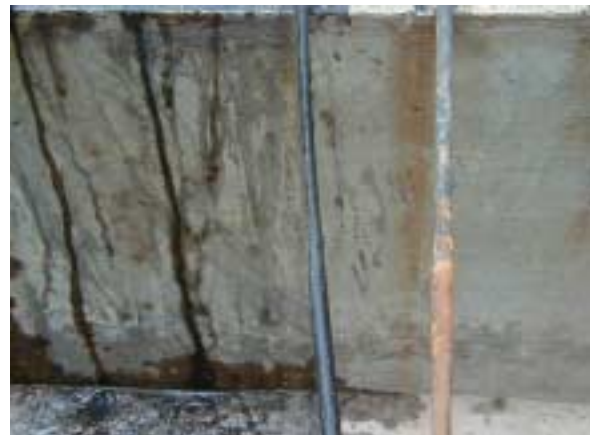
4. Ferrous hydroxide Sedimentation at No. 175
