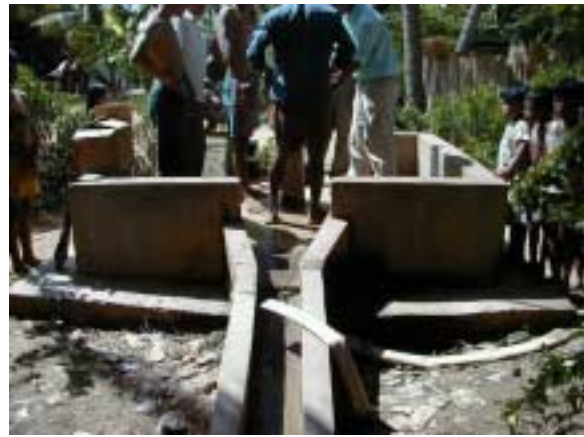
8. Damaged by settlement at No.288
