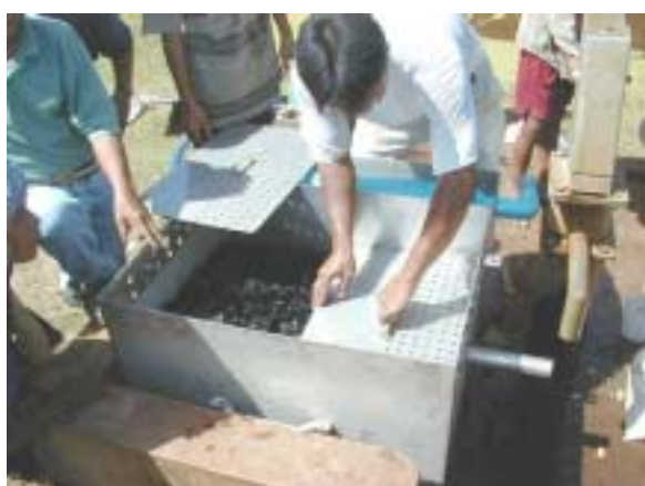
11. Putting on the perforated plate
