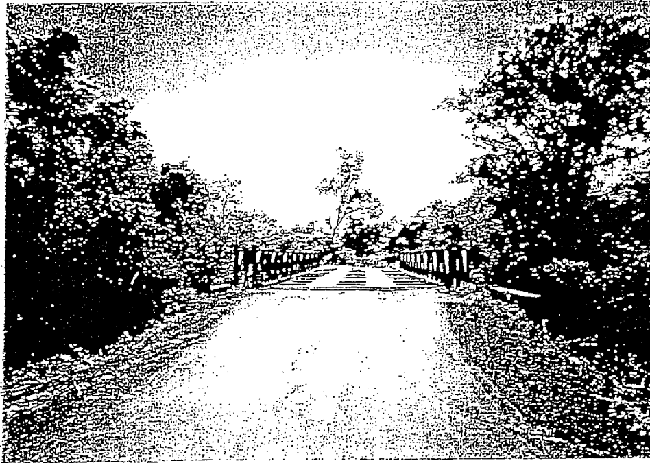
Figure. 3 General view of Bridge no.1
