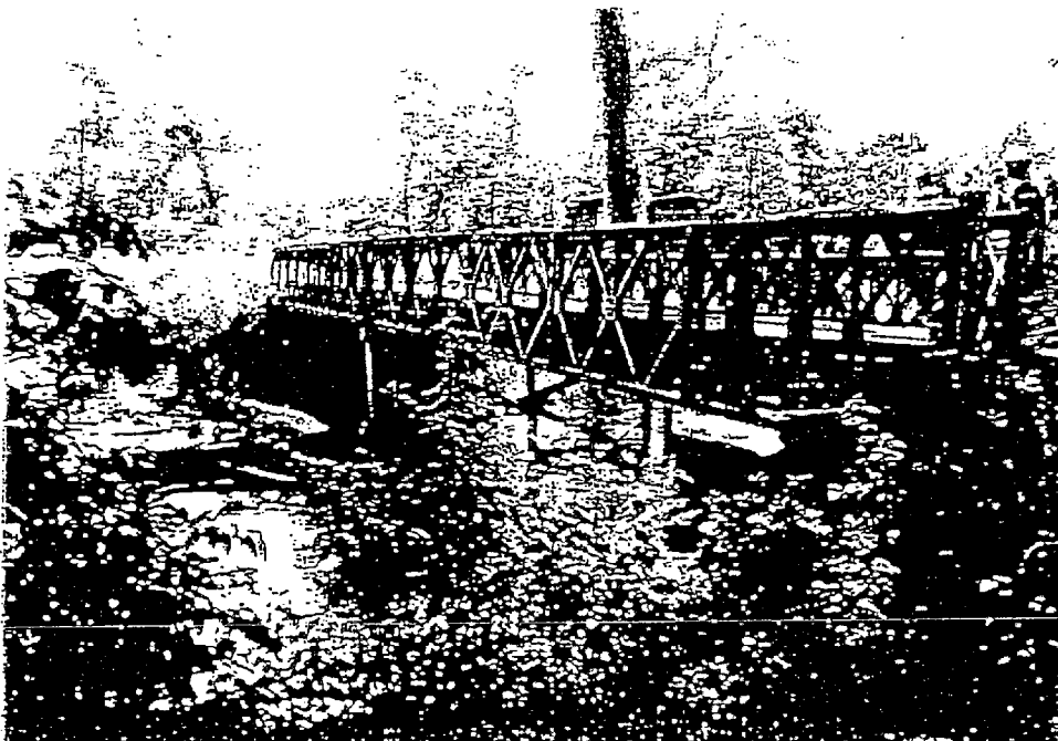
Figure. 27 General view of Bridge no.13
