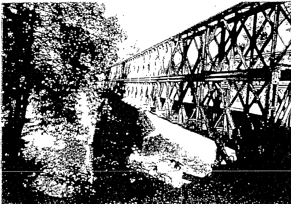
Figure. 31 General view of Bridge no.15
