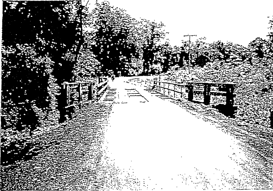
Figure. 11 General view of Bridge no.5
