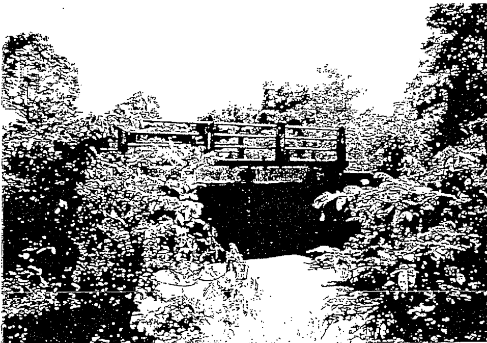
Figure. 20 General view of Bridge no.9
