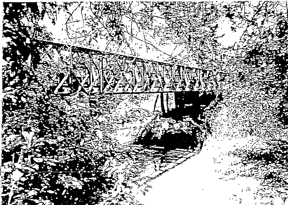
Figure. 4 General view of Bridge no.1
