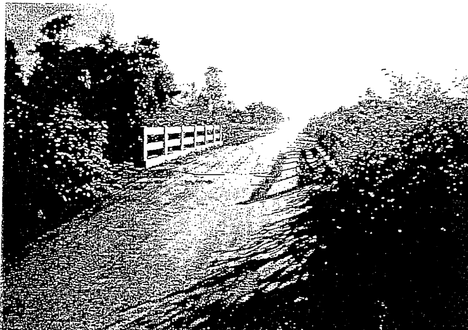
Figure. 38 General view of Bridge no.19
