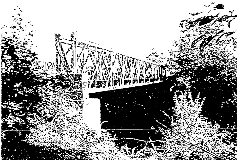
Figure. 35 General view of Bridge no.17
