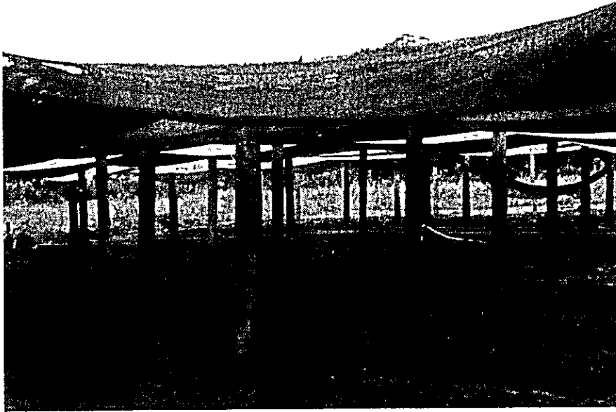
Photo Number 7 Sun covering (high covering)
