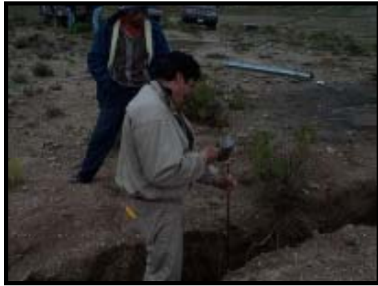
(b) Grounding work
