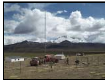
Wind Monitoring Tower of Caripe
