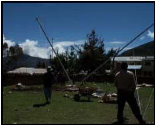
(c) Monitoring tower erection
