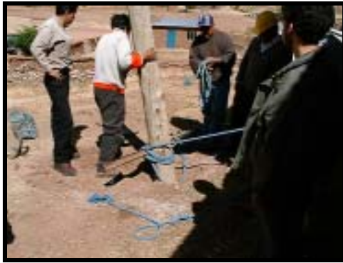
Removal of the installed PV System
