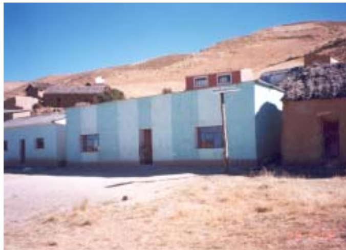
PV system at school in Achaya community
