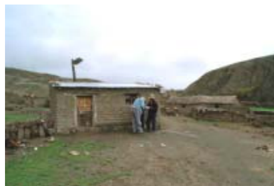
A house with a PV system
