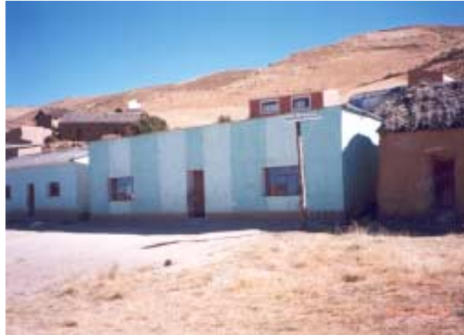
PV system at school in Achaya community
