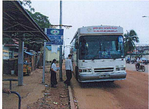
Bus Stop and Bus Shelter
