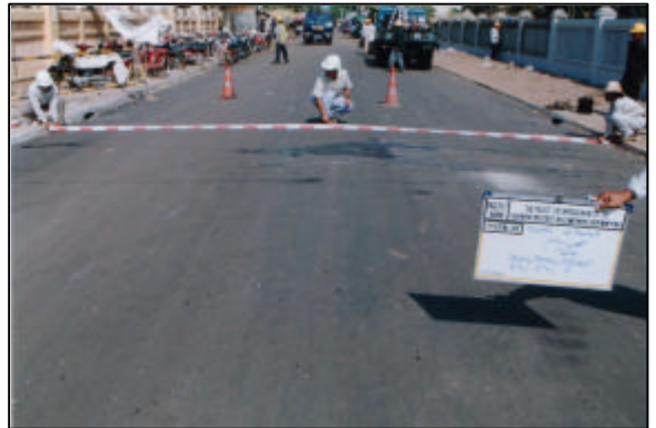
St.105 after Improvement
