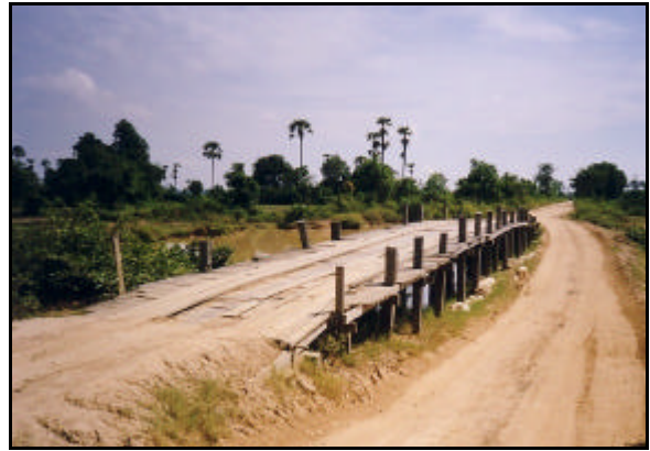
Timber Bridge on Suburban Road
