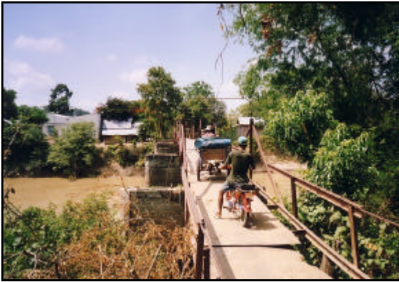
Narrow Bridge on Suburban Road
