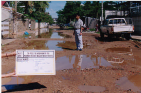
St.105 before Improvement
