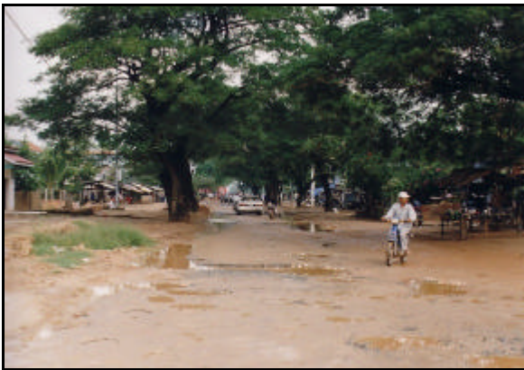
Suburban Road with Poor Pavement Condition
