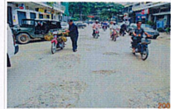
Road in Bad Condition
