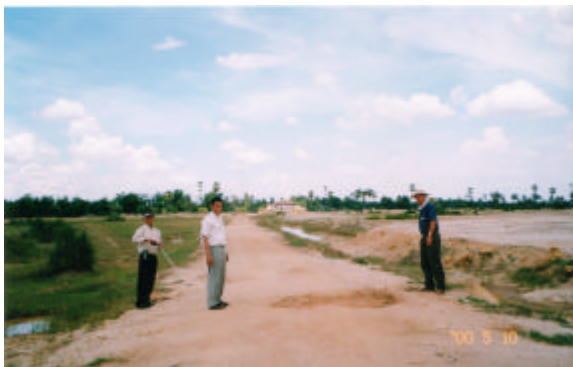
On-going Development in Suburban Area
