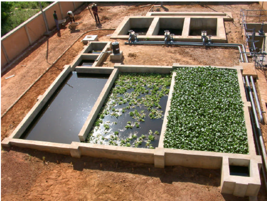
ECO-POND AND SLUDGE DRYING BED
