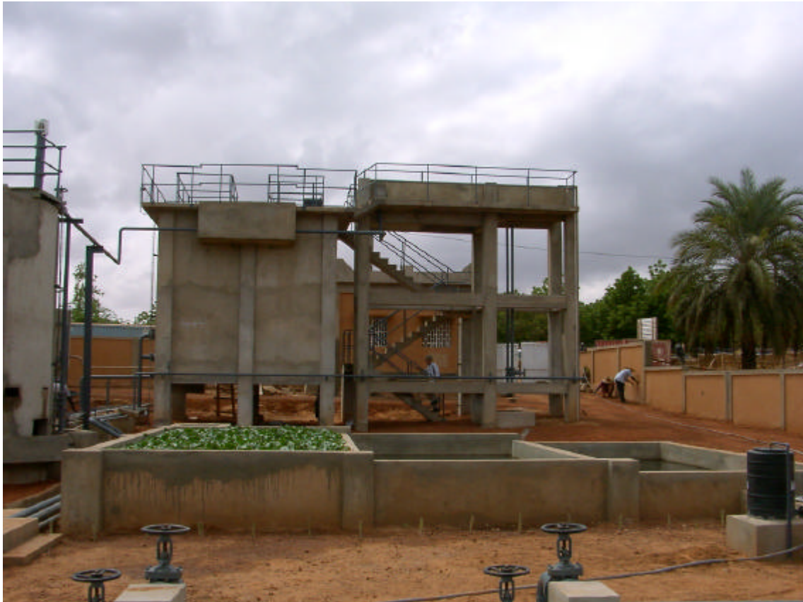
UASB REACTOR AND BIO-TOWER
