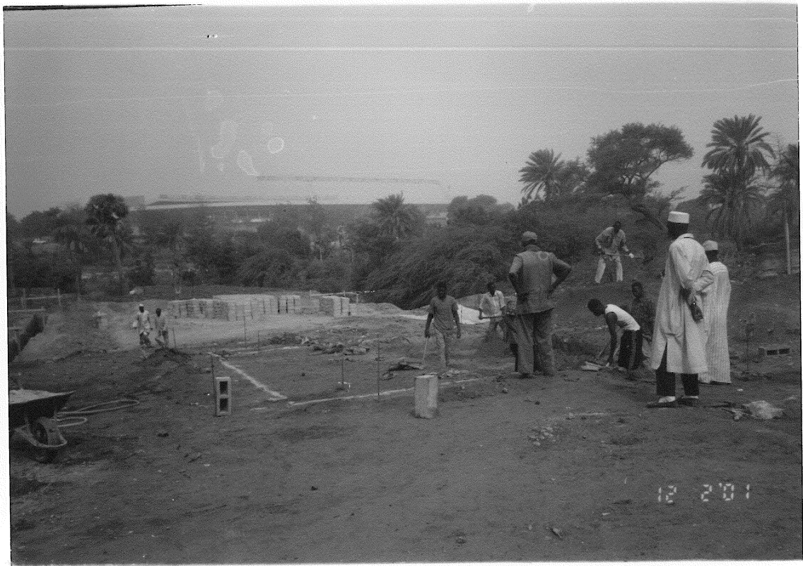
Earth work of main building of UASB
