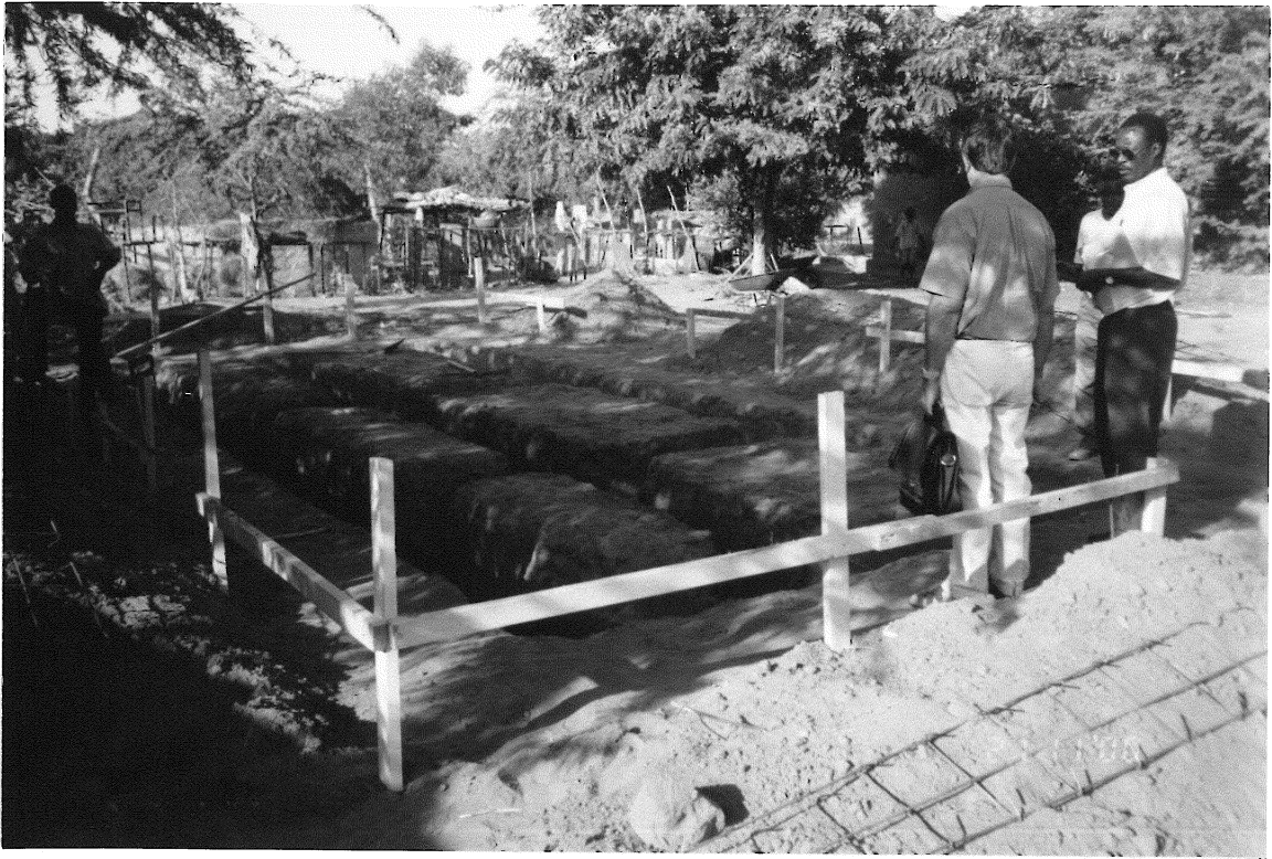
Foundation work of toilet
