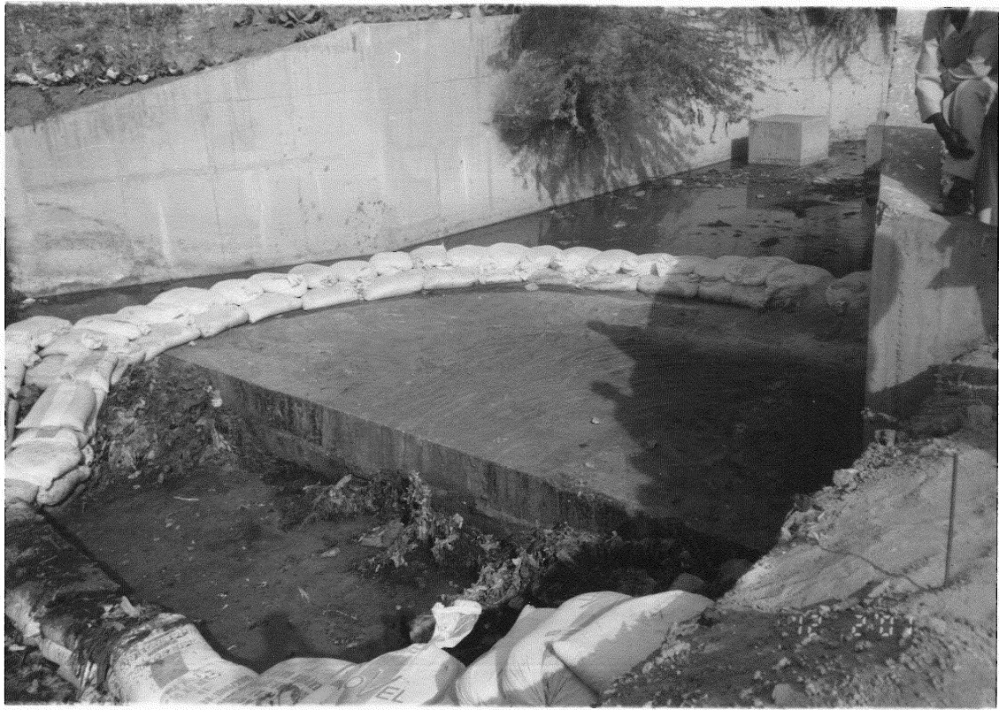
Diversion work of inlet work of UASB
