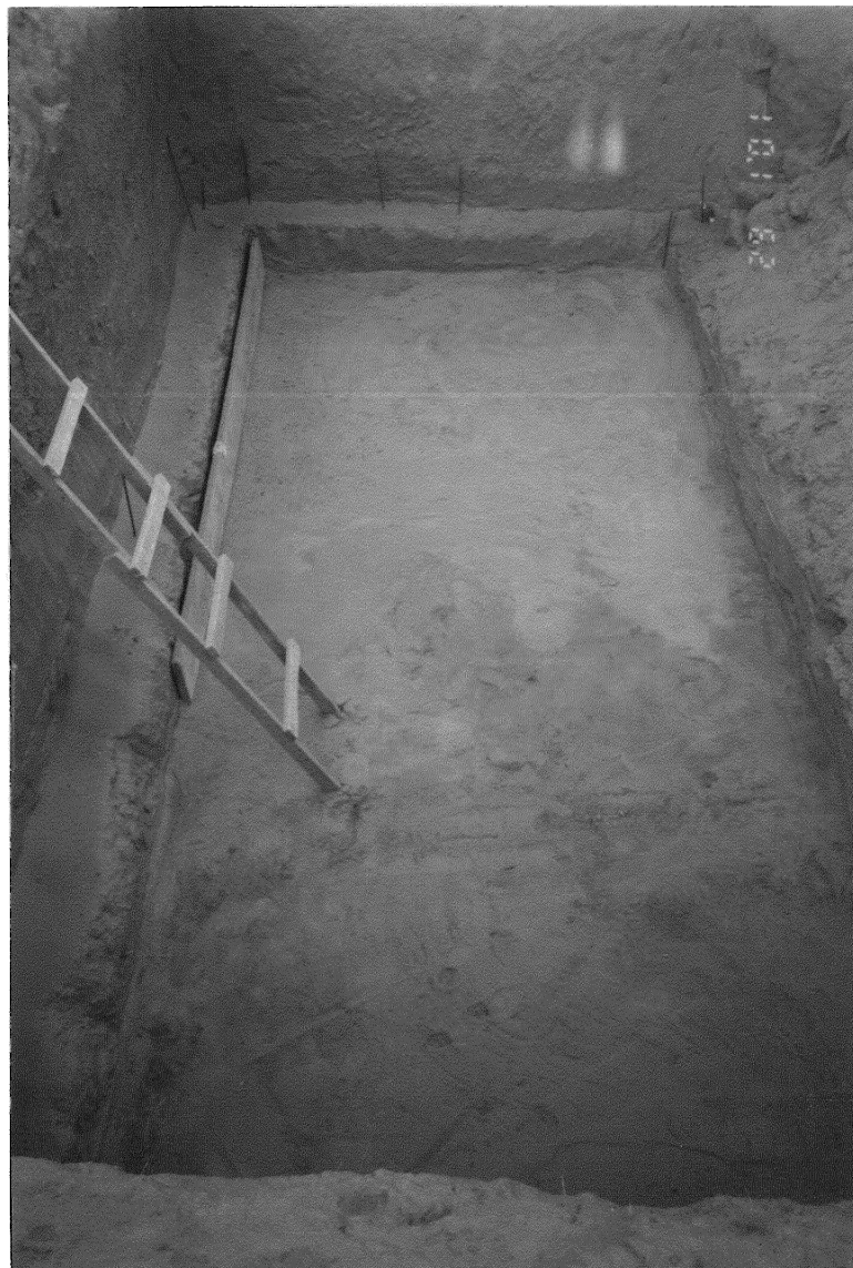
Earth work for Jyokaso
