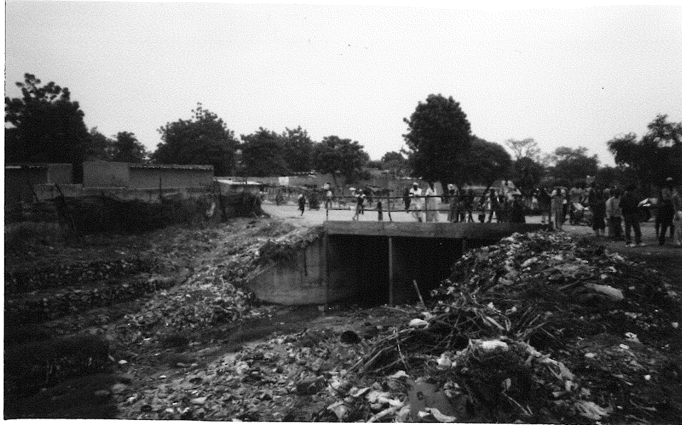
Waste dumped near road crossing of Gountry Yena River
