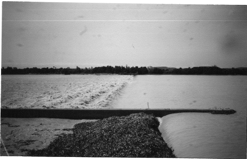
Intake weir at Goudel Water Treatment Plant
