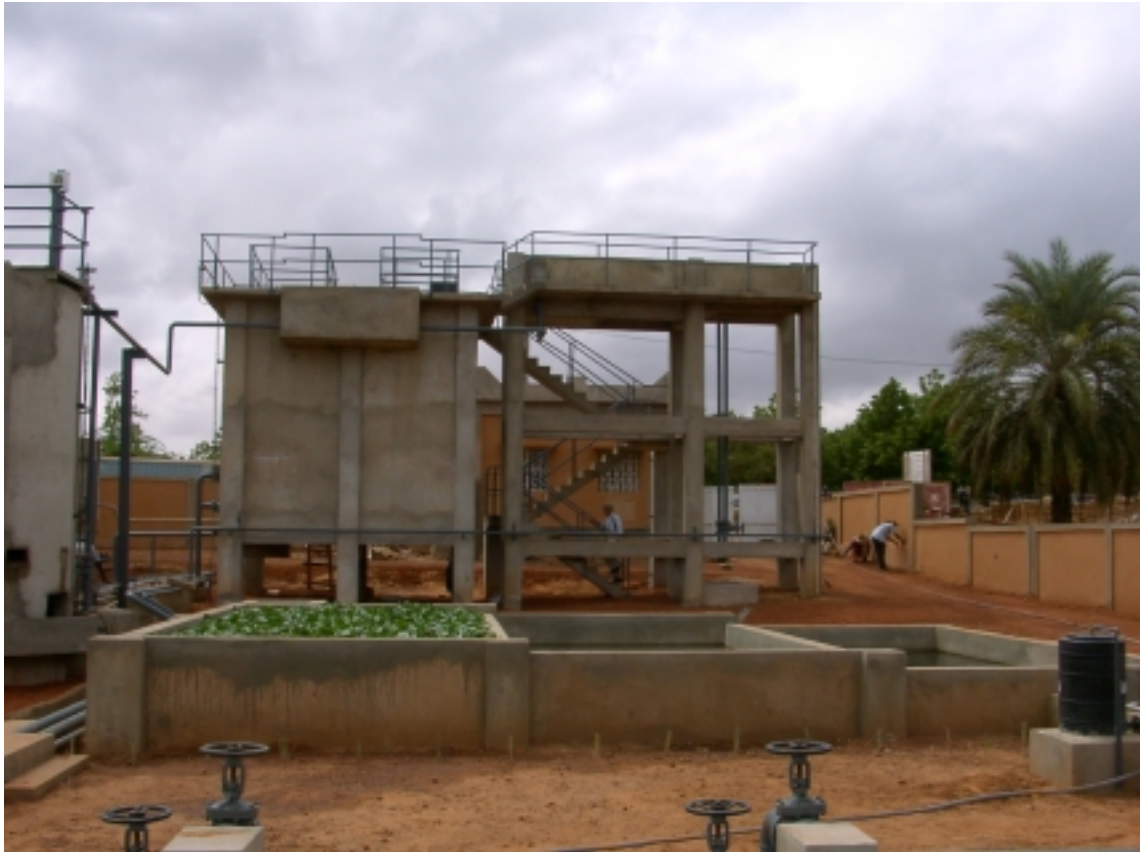
UASB REACTOR AND BIO-TOWER
