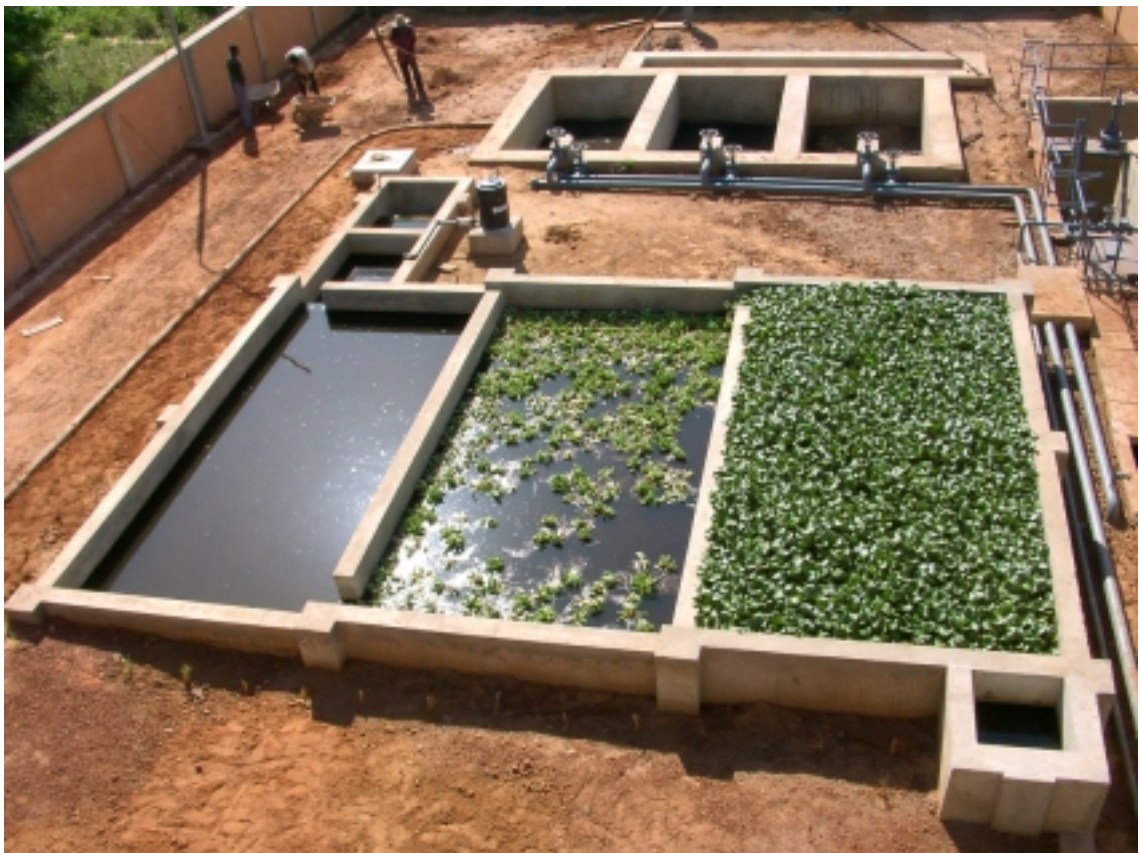
ECO-POND AND SLUDGE DRYING BED
