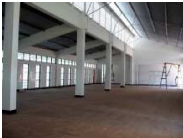
New library under repair work : 100 seats and 34,000 books (expected)
