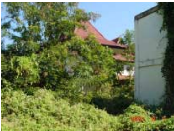
Building C Exterior View
