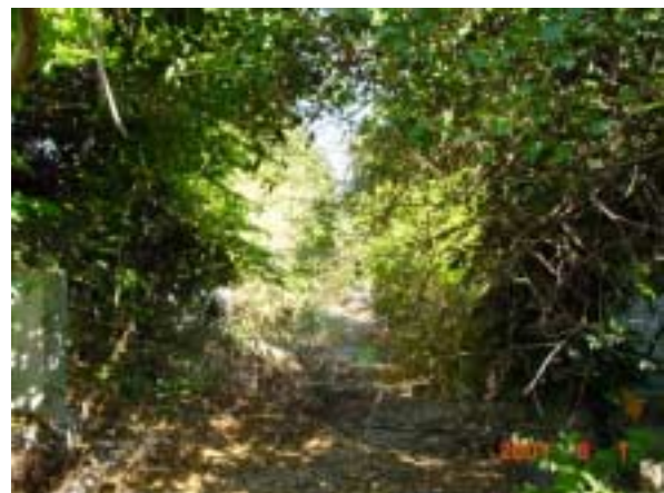
Road is covered by bushes.
