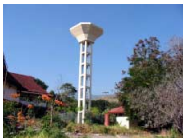
Tower of the elevated water tank
