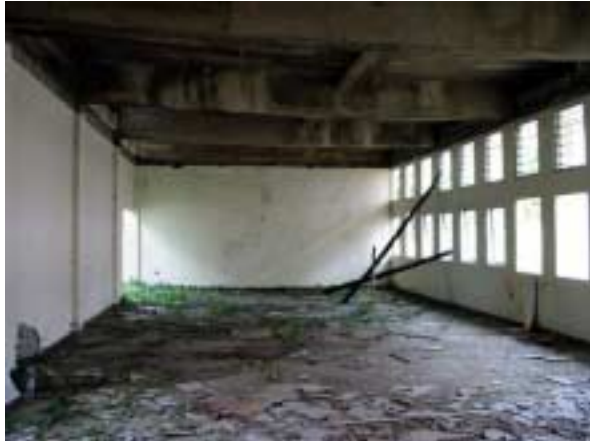
Classroom 1-3: Ceiling and floor tiles are removed
