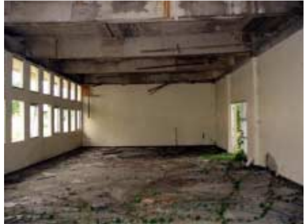
Classroom 1-3 : Ceiling, floor tiles and ALM sash are removed.
