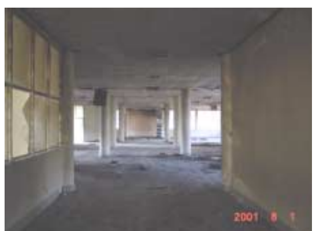
2 nd floor : Interior view
