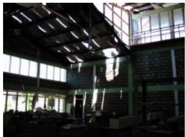
Workshop Interior View : Ceiling and roof were damaged by fire.
