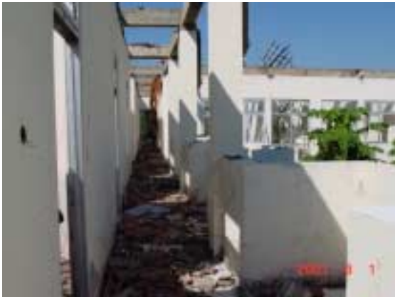
Building B 2 nd Floor corridor
