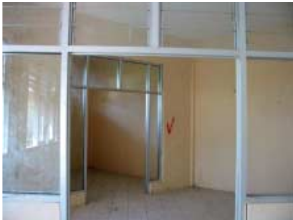
Laboratory annex room : Door panels are removed
