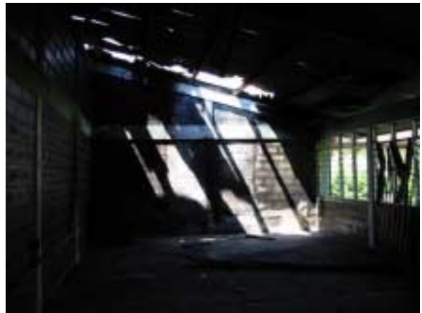
Lower part of Workshop : Roof was broken by fire.
