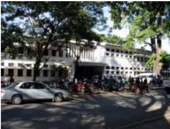
Entrance of the Main building
