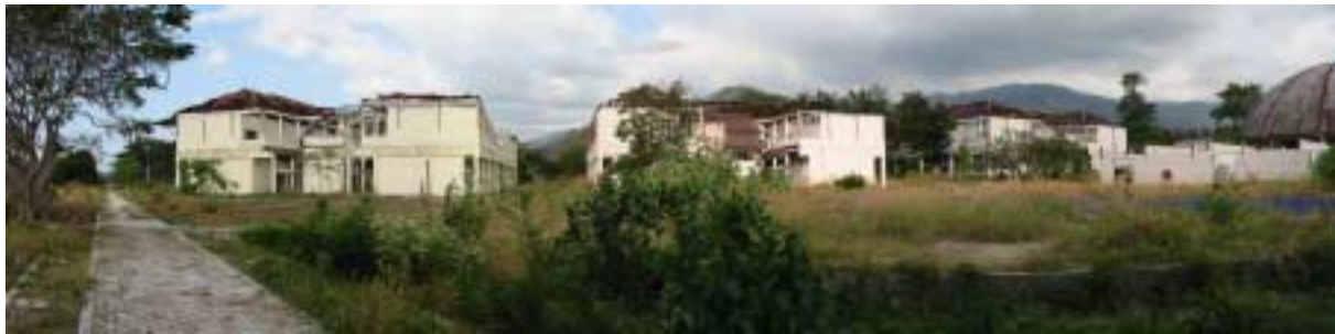
Panorama view of Lecture building A,B and C.
