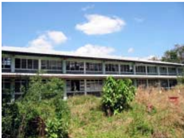
Exterior View : Aluminum sashes were broken.
