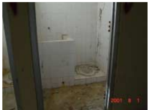
Toilet and shower booth
