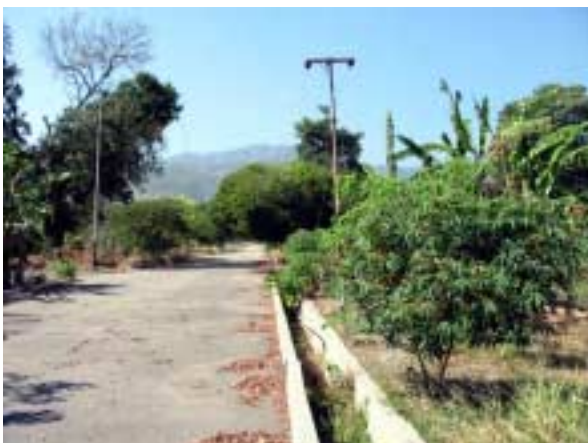
Secondary cable was cut off in residential zone
