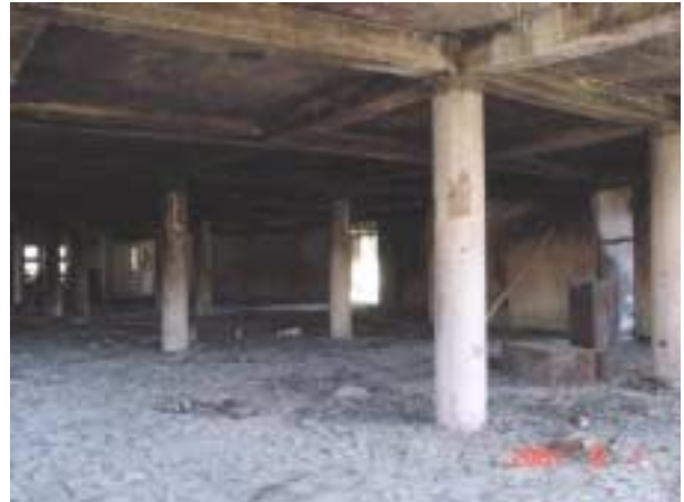
1 st floor : Interior view 2
