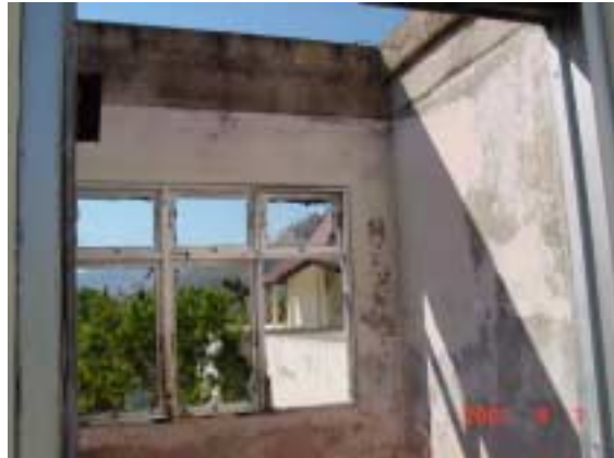
Building B Bed Room: Interior view
