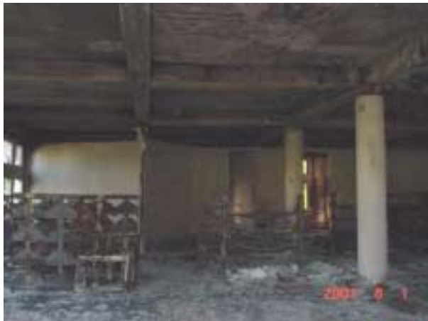
1 st floor : Interior view 1
