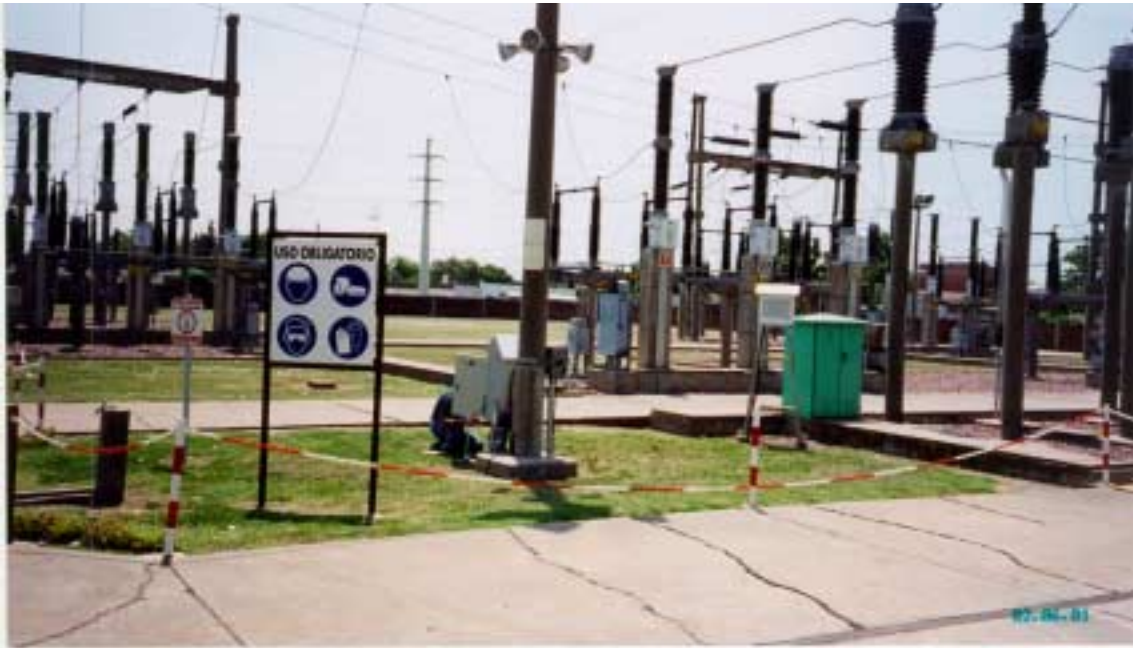
TRANSIBA (Transforming station) in the San Nicolas Area
