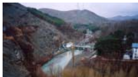
Existing Bileghan Intake from where Karaj dam water is Conveyed to Tehran City
