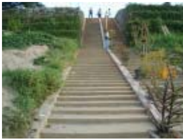
Existing Slope Staff Gauge
