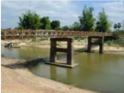
Proposed Site of Slope Staff Gauge Station
