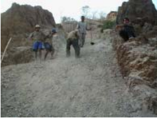
Xeingkok slope gauge station (Luang Namtha Province)
