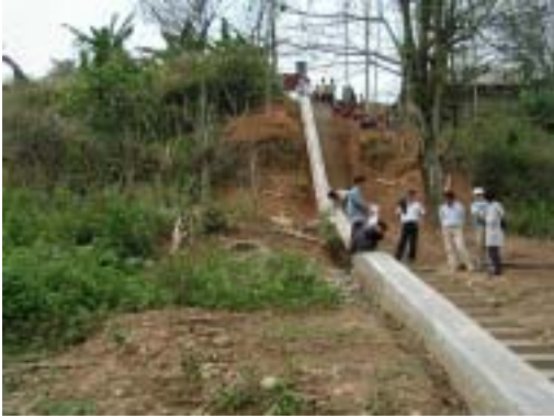
Naluang slope gauge station (Xai Songbung Special Zone)
