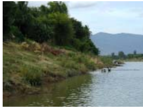
View of Slope Staff Gauge Station
