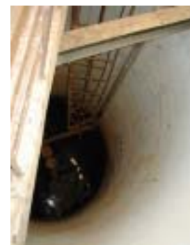
Inside View of Water Supply Tower
