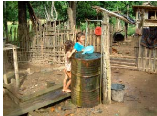
Rural Water Supply Facilities (Louangphrabang Province)
