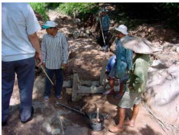
Canal Construction by Farmers' Participation (Oudomxai Province)
