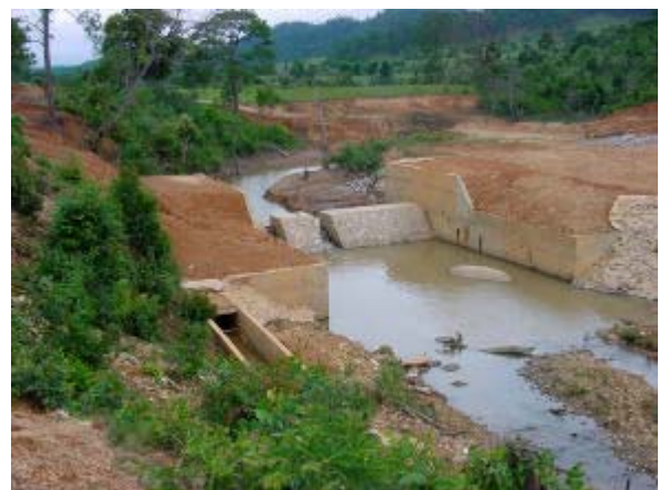
Headworks constructed by Community Managed Irrigation Sector Project (CMISP) (Xiangkhouang Province)
