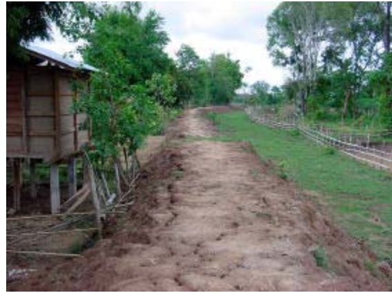
Flood Protection Dike (Savannakhet Province)
