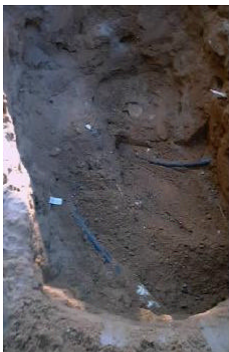
Photo Trial pitting, encountered with Cables and Groundwater
