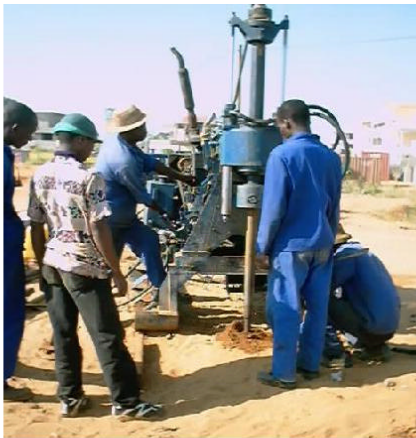
Photo Drilling Rig at Borehole No.2 with Close-up View
