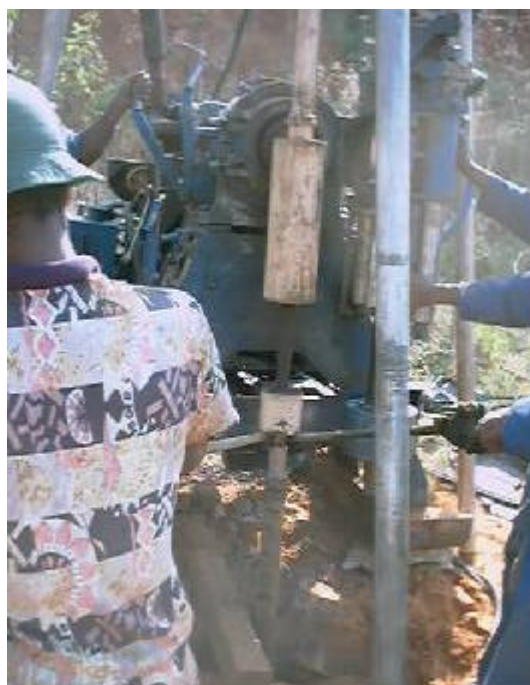
Photo Drilling at Borehole No.3 and SPT Scene
