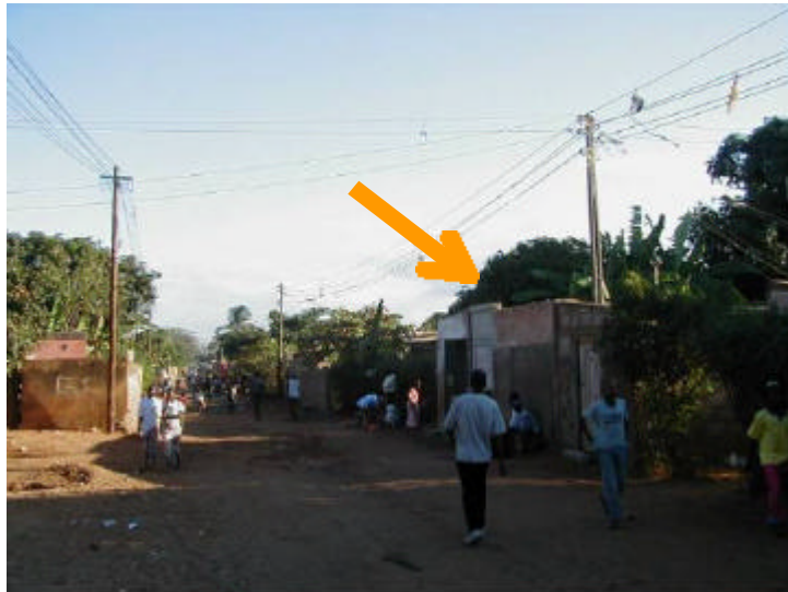
Photo 15.7.1 Illegal Housing on Collector Roads
