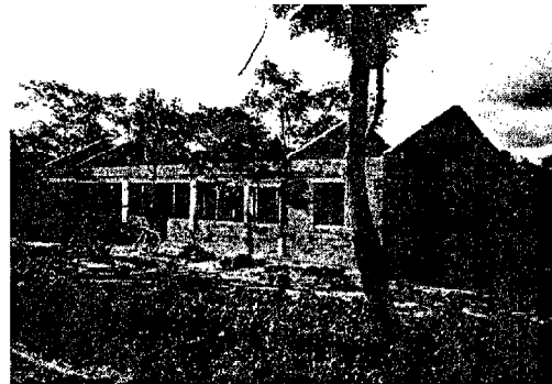
Construction of Community hall
