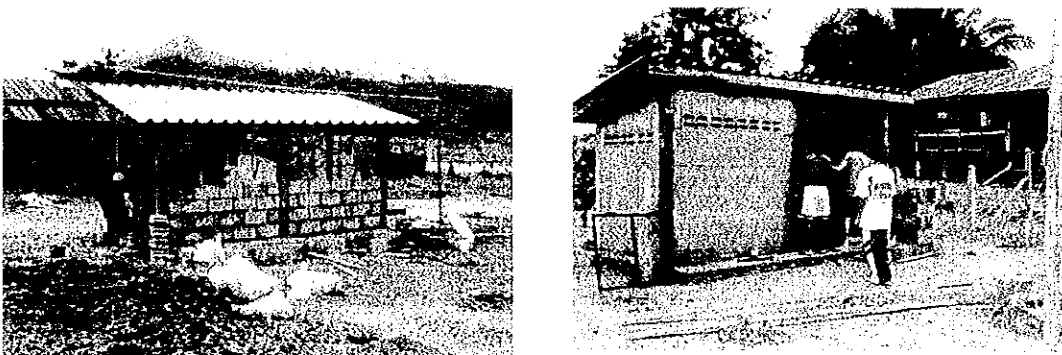
Figure 5-4-6 Battery charge room
