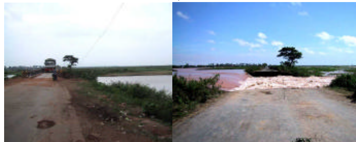
National Road 1 Damaged by flood (Sep. '00) and Bridge spanned the damage (Kandal province)
