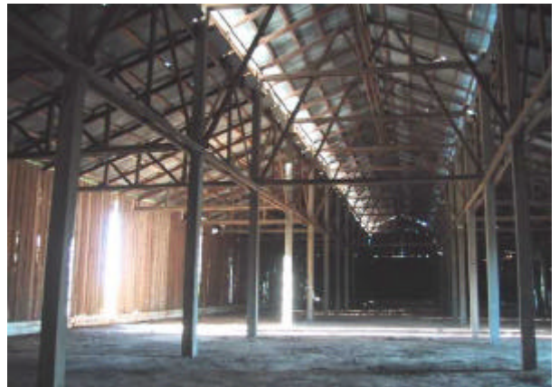
same as left (inside of warehouse)
