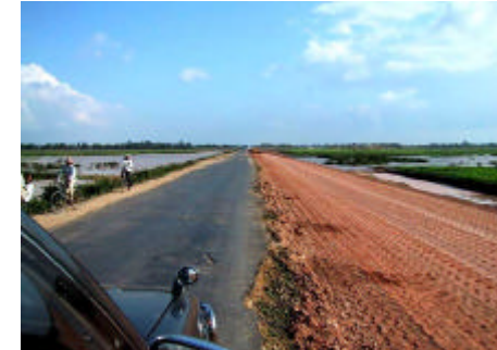
National Road 1 Rehabilitation work assisted by ADB (Svay Rieng province)
