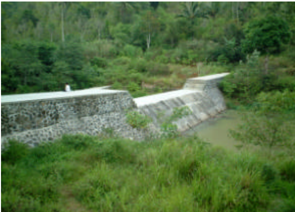
Dam Pengendali (Check Dam) Batu Kali (Toulinag Oki)
