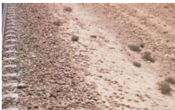
Photo 3.3.3 Slope of Embankment
