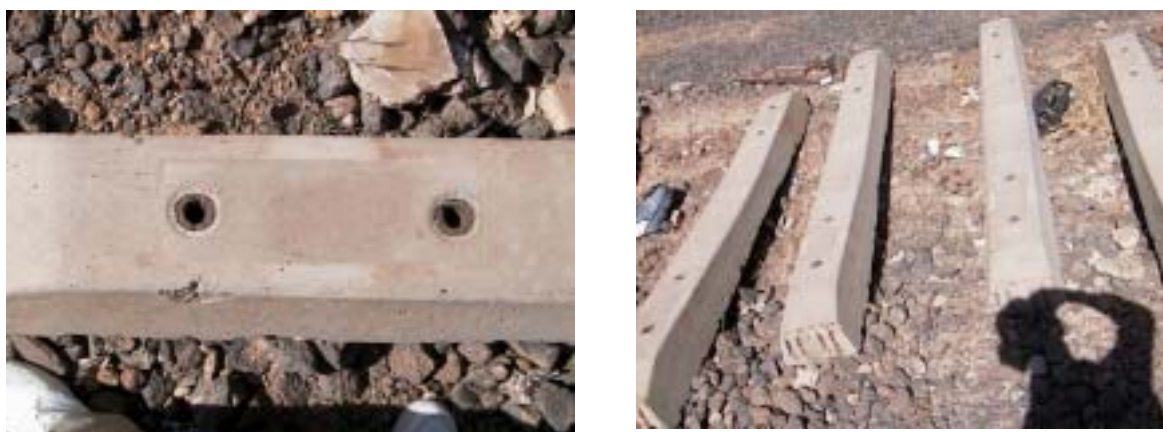
Photo 3.3.2 Concrete Sleeper and Wooden Tie Plug
