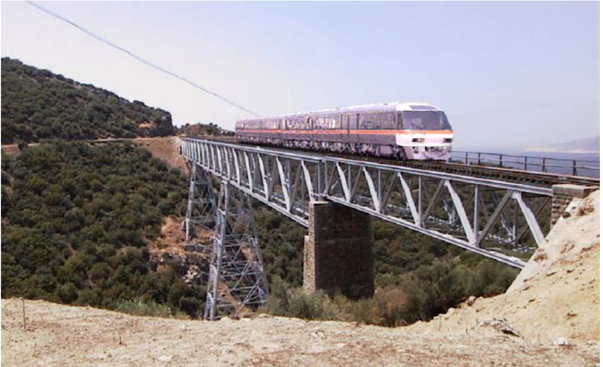
Diesel Car Train Passing through the Bridge
