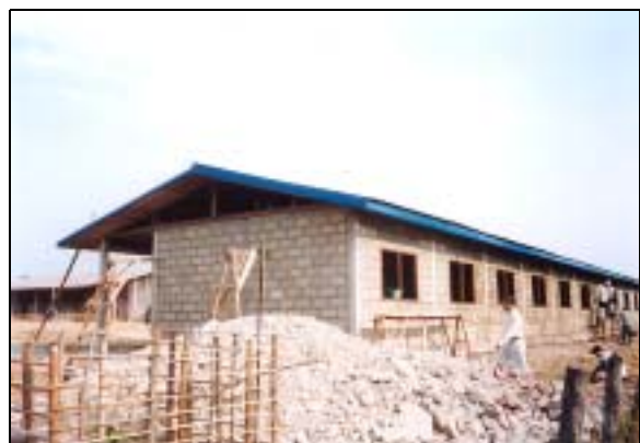
Photo 24 New school under Construction, donated by Japan's NGO (Atsaphangthong, Savannakhet)
