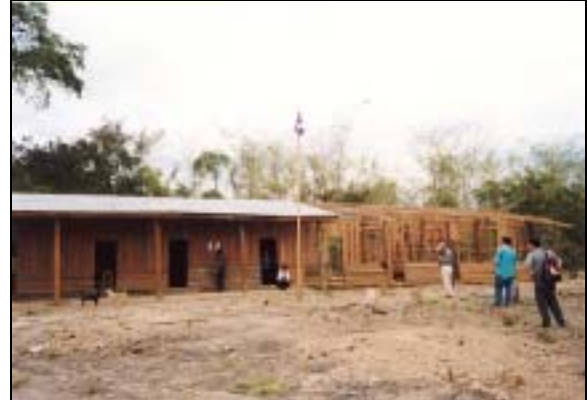
Photo 8 School in Ban Panam (Mahaxay, Khammouan)
