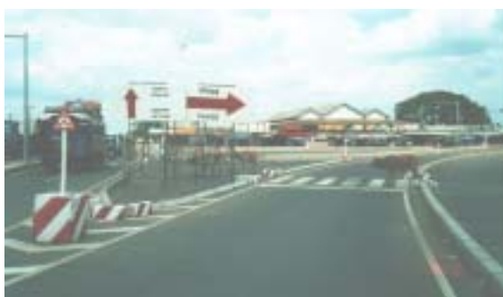
Figure 7. 8 Completed Section of Route 9 at Xeno
