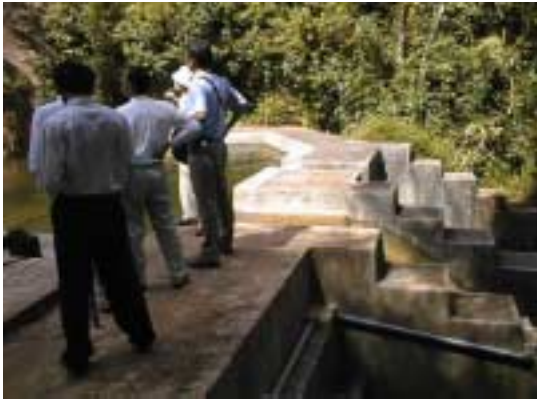
Existing intake weir
