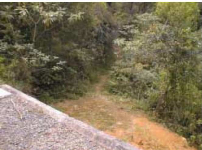
New Water Field Reservoir
