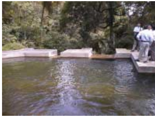
View from upstream of intake weir
