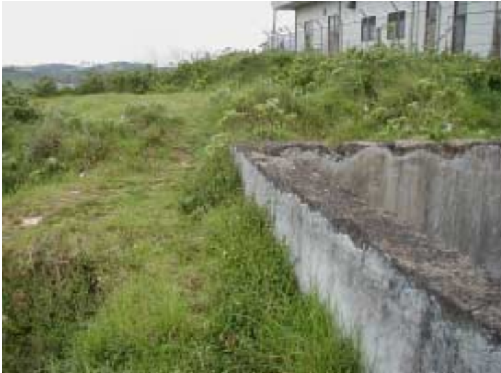
Concrete structure is abandoned reservoir backyard is construction site
