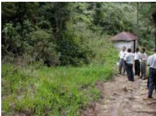
Construction site of elevated tank (left side)
