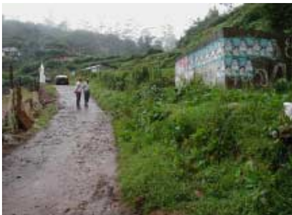
Access road to the construction site
