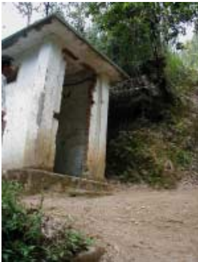
Abandoned guards house New reservoir will be constructed here
