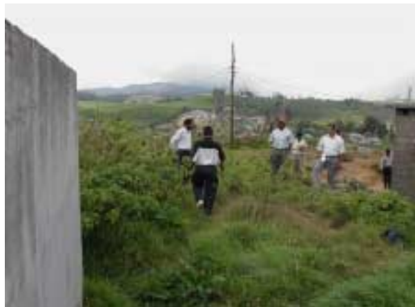
Construction site of reservoir Left concrete structure is existing reservoir
