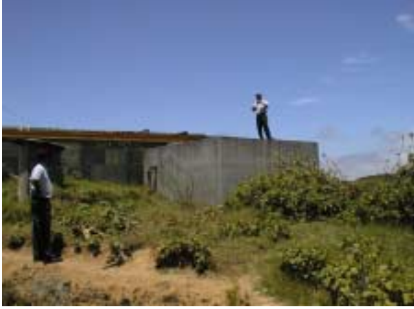
Existing reservoir Construction site is in front
