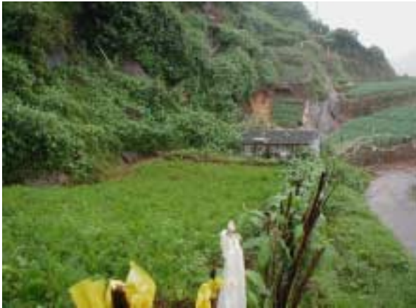
Construction site of new reservoir, concrete structure is existing reservoir
