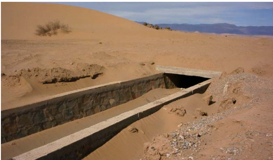
Photo No.42 Buried Canal Line Sandy Soil
