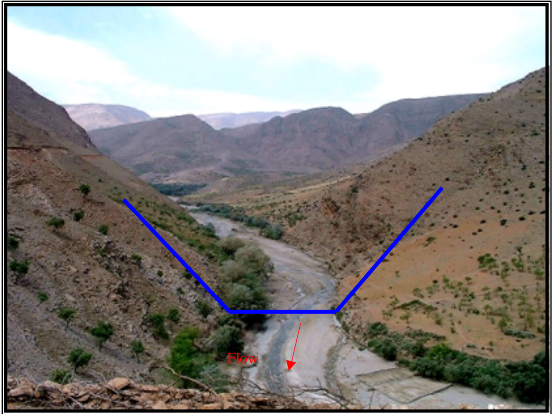
Dam Axis of Taskourt Site
