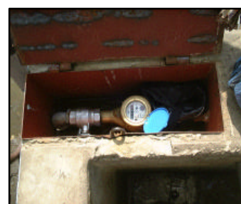
Water Meter installed on the Top of Tap Stand, Chibolya
