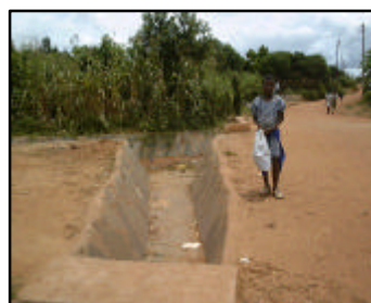
Stone Pitching in Drain of Ng'ombe Pilot Project
