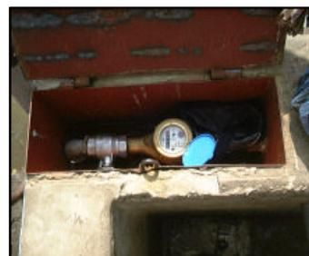
Water Meter installed on the Top of
