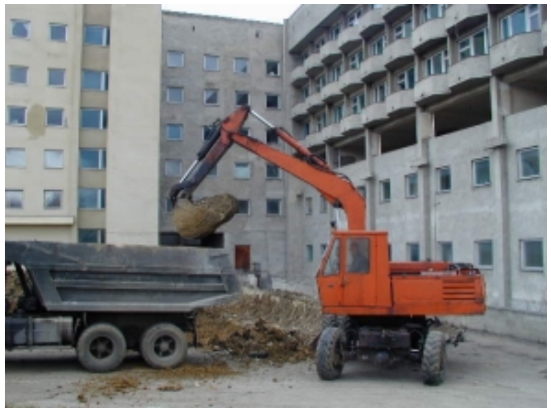
Renovation work of the hospital (Prof. O. Gudushauri General Hospital)
