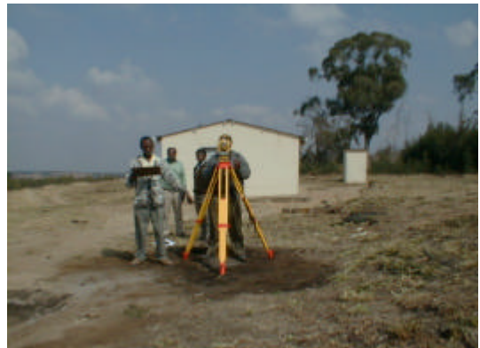
Measurement of elements of eccentricity using a TotalStation
