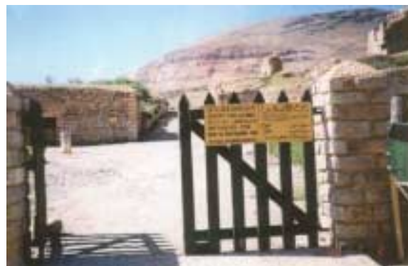
Entrance notice board giving a very poor impression. Some symbolic ornamentation can be applied.
