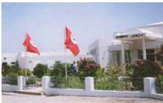
Entrance to Chemtou Museum. In the left, a sign for toilet. This museum was a good attempt with German assistance. However very few visitors are counted.
