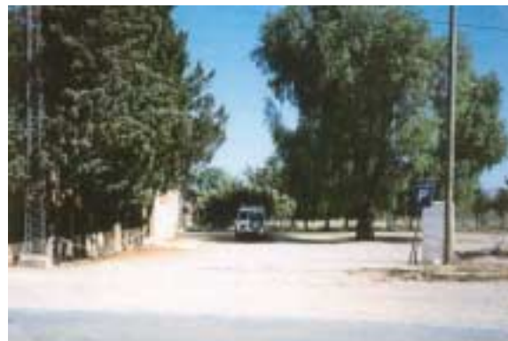
Parking. Not paved nor line-marked. Should be improved with landscaping.
