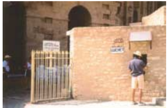
Ticket booth and entrance. Sign panel can be improved together with the ornamentation of the entrance.
