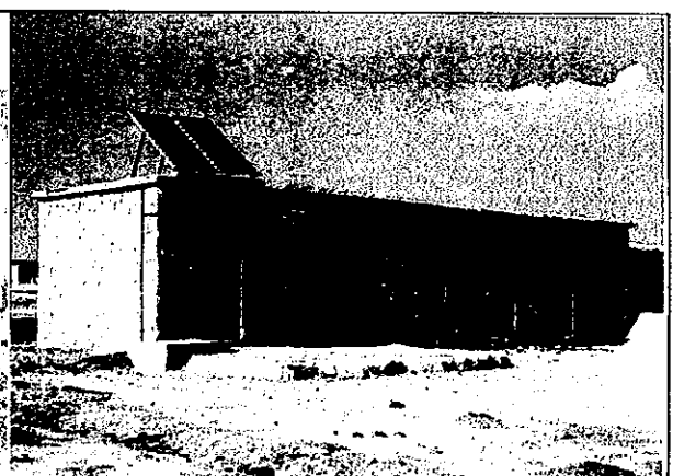
View of PV array (Roof mount type)
