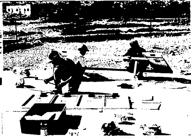
Interconnection among PV module July/1997 (Fedre)
