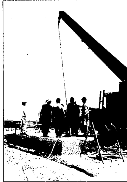
Installation of water pump July/1998
