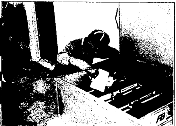
Interconnection among battery July/1998
