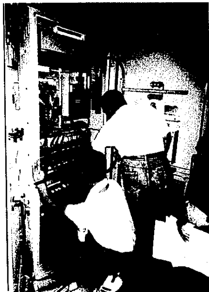
Inspection of main equipment July/1998
